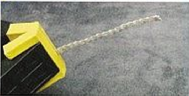
Figure 4 Cut the remaining wires blunt to the wrap.
